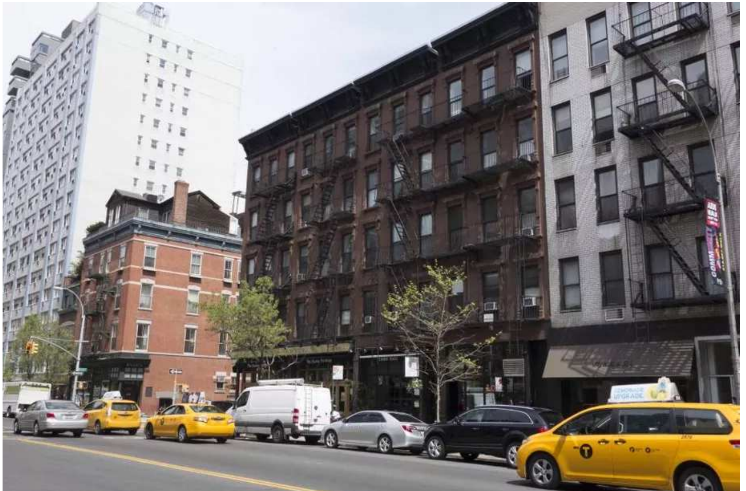
202 East 13th Street, one of the buildings owned by Steve Croman's 9300 Realty Nicholas Strini/PropertyShark
