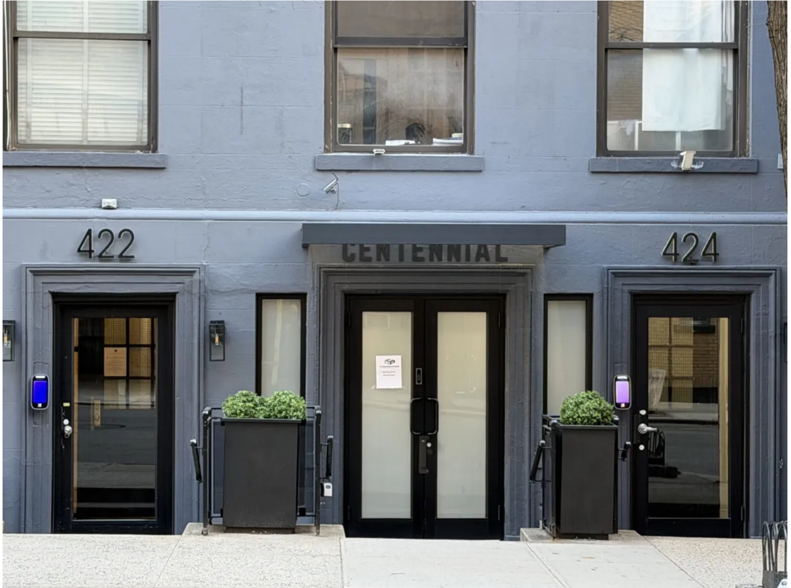
Centennial Properties offices on W51st Street between 9/10th Avenues in Hell's Kitchen. Photo: Phil O'Brien
