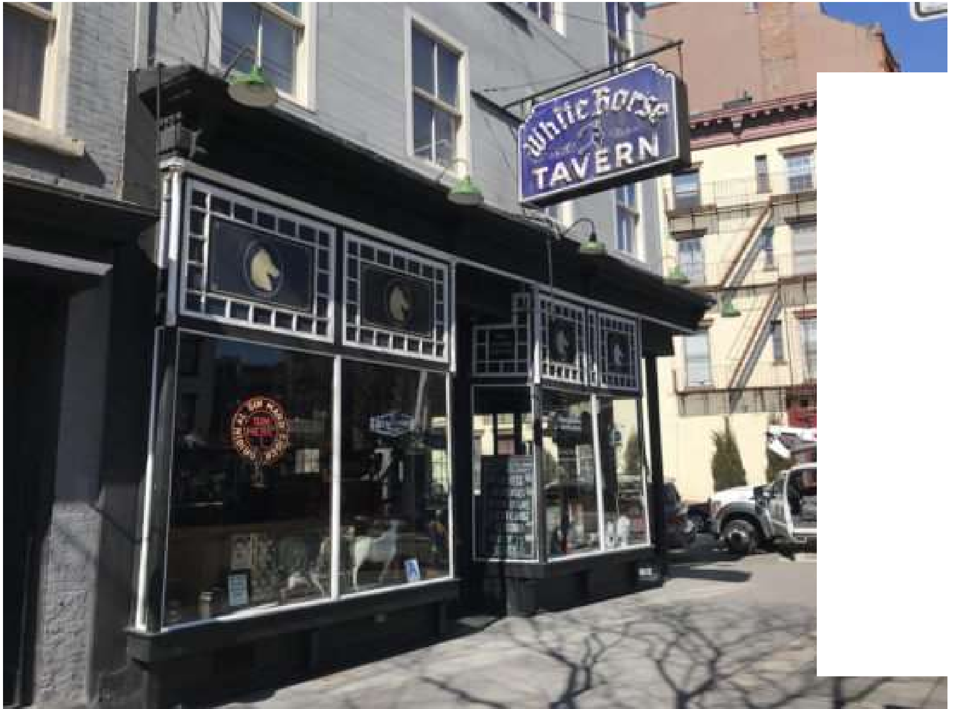
The exterior of the White Horse Tavern, at Hudson and W. 11th Sts., is landmarked as part of the Greenwich Village Historic District. (Photo by Gabe Herman)
