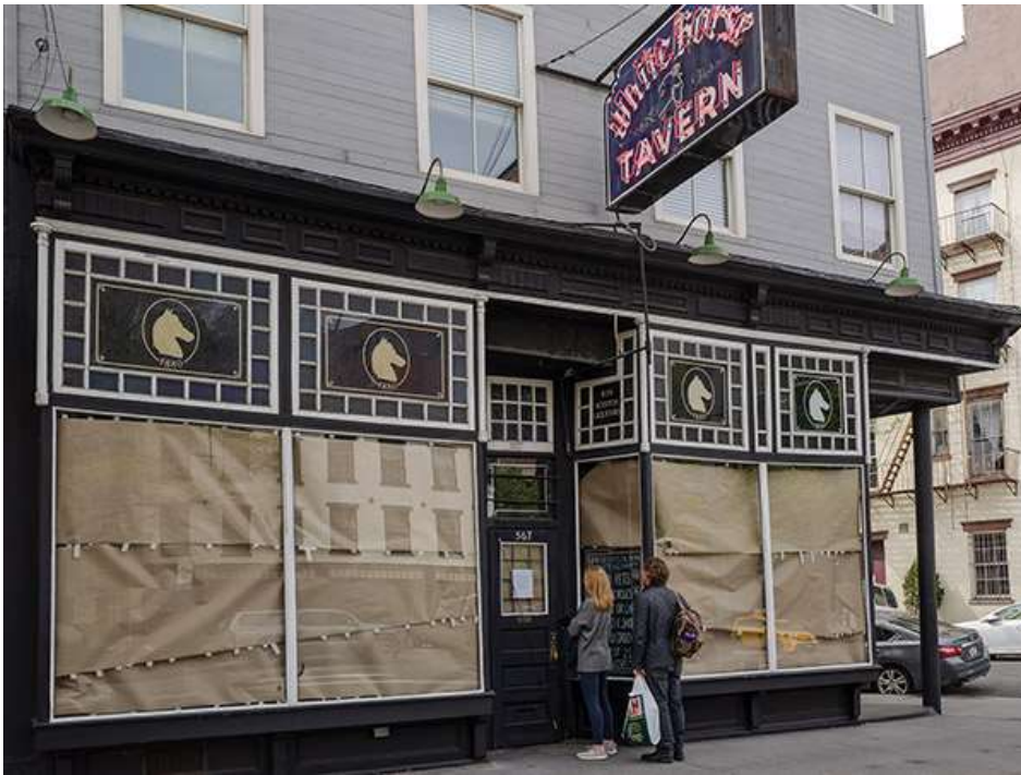
WHITE HORSE CLOSED FOR PIZZA? West Villagers await with apprehension the refurbishing by noted Pizza restaurant owner. Photo by Chris Manis.
